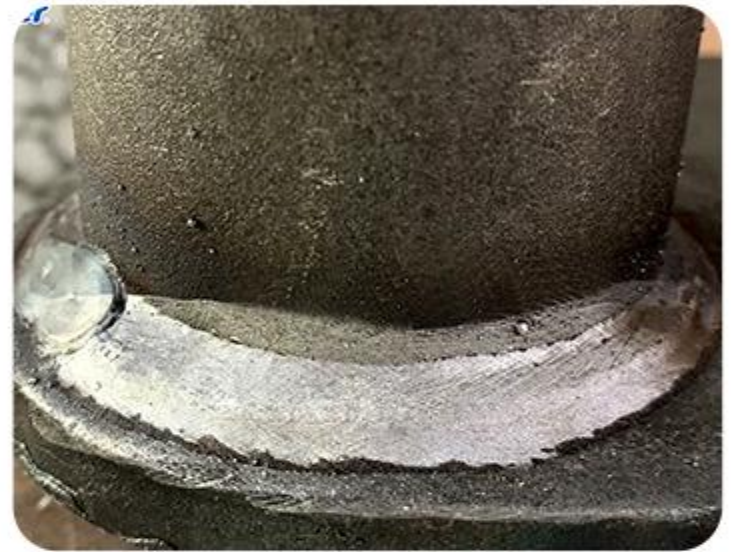
Weld Seam Cleaning
